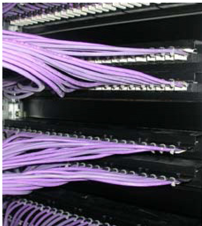
Rear of high density patching facility
